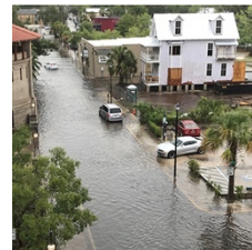
Figure 52. Flooding – St. Augustine
