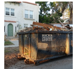
Figure 58. Other – Removal of Historic Building Materials, St. Augustine
