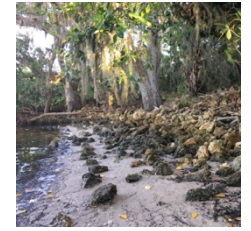
Figure 24. Other: Mitigation Strategy, Shoreline Revetment (Emerson Point Stable)
