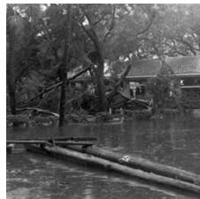
Figure 51. Wind and Storm Damage Plaza de la Constitucion (Florida Memory)
