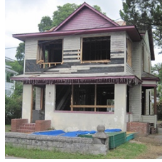
Figure 61. Other – Removal of Significant Building Elements, St. Augustine
